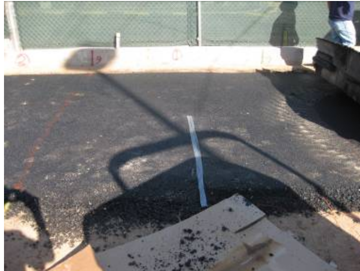
Figure C.7 – Installation of Thermocouple on Asphalt Base
