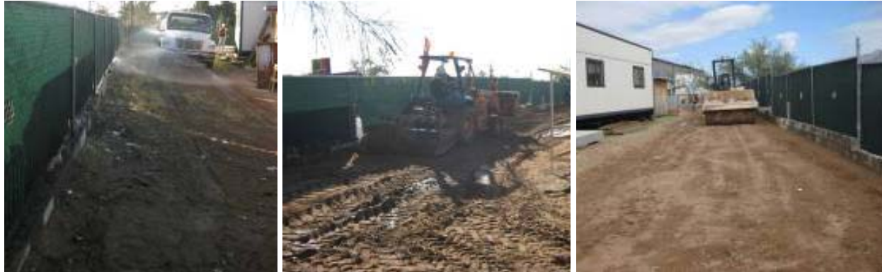
Figure C.4 – Preparation of Subgrade
